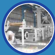
Aluminum Extrusion Plant
